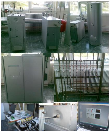
Fig. 3. The laboratory of Cogeneration Energy Based on Solid Biomass; a – solid biomass heating system; b – air – water heating system; c – data acquisition system for biomass heating system.
